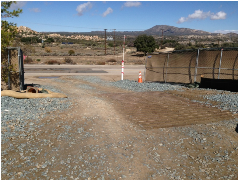
Photo 2: In accordance with the Dust Control Plan (Mitigation Measure BIO-4A), rattle plates have been installed at the Boulevard Substation where the dirt access road intersects paved surfaces associated with Old Highway 80.
